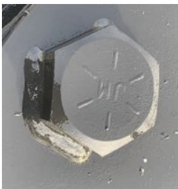
FIGURE 4.7A BOLT HEAD BEAD WELD & ASSEMBLY
